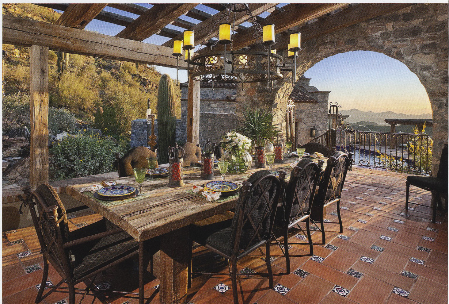
Rough-hewn beams form a pergola over the home's open-air dining patio. Flooring of Spanish Cotto tiles in a basket-weave pattern is accented with Mexican tiles.
